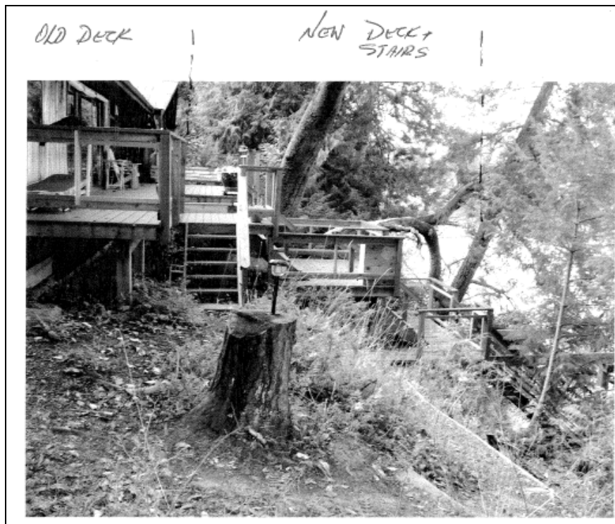
Figure 1 Image showing deck expansion and stairs
