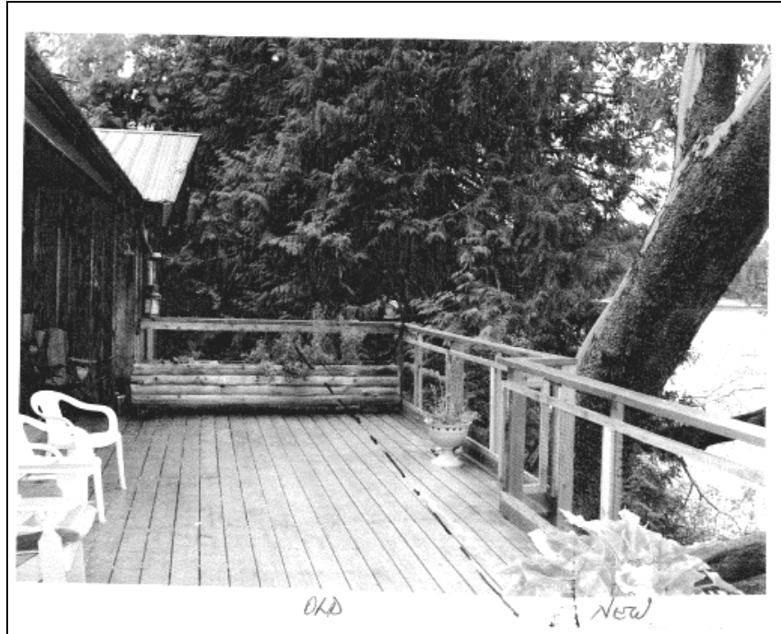
Figure 2 Image showing deck expansion
