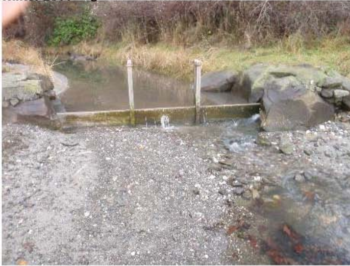
1.) Deacon Creek weir at intertidal boundary
