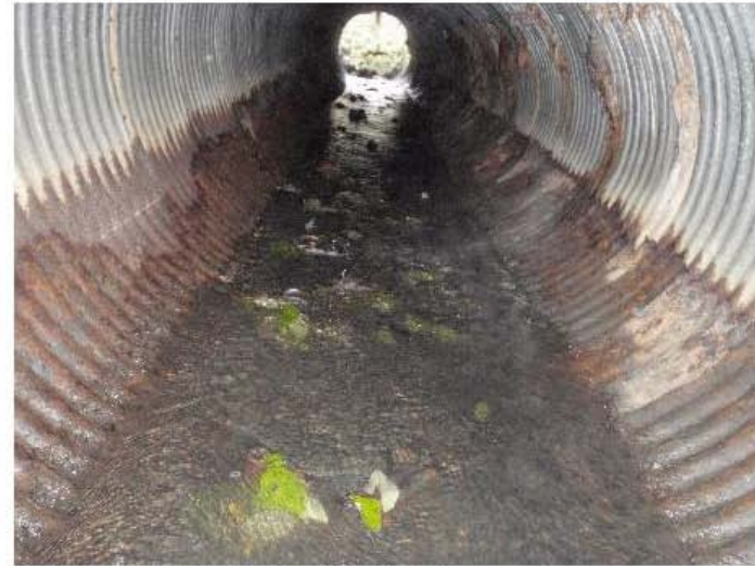
3.) Culvert below Village Bay Road
