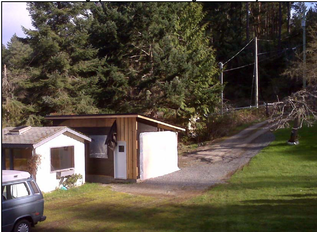
Photograph 1: Location of Garage and Driveway
