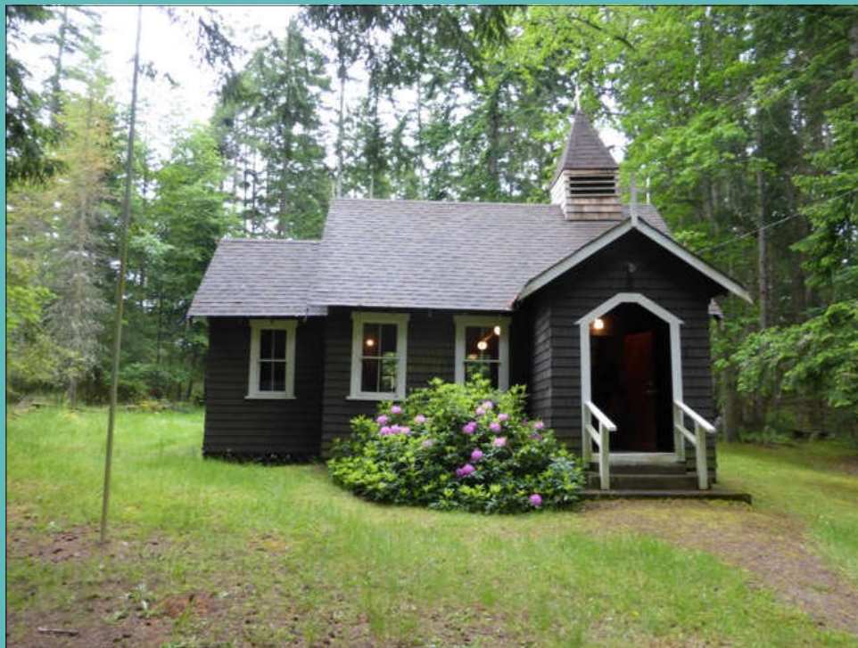
South elevation of Church of the Good Shepherd showing gable entryway.
